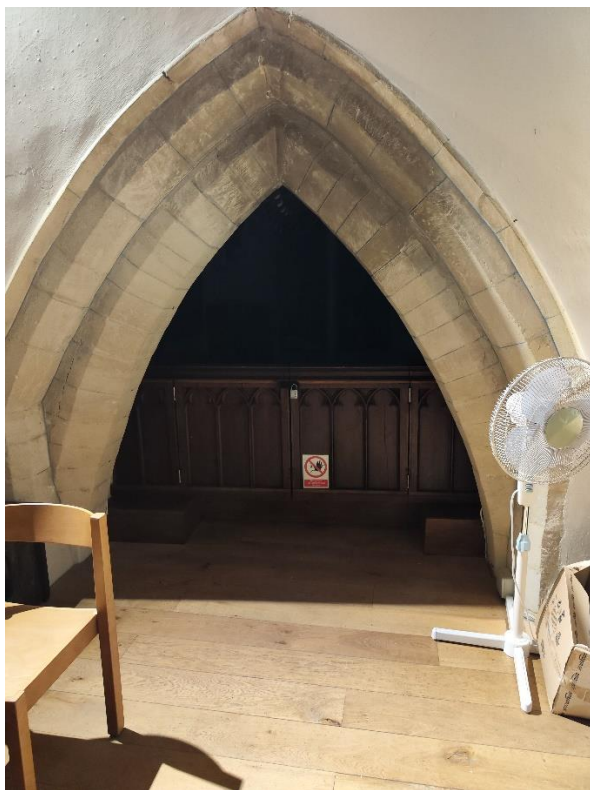
Figure 2 Bell ringing chamber with half gates fitted in the arch.
